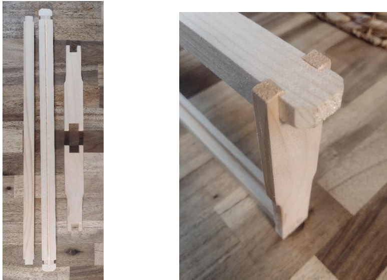
Figure 2 Frame Pieces and Assembled Hoffman Style End Bar
